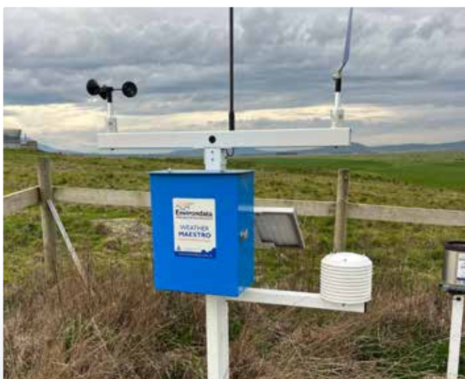
Sensor Shelter on a typical 2 metre Weather Station
